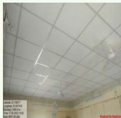
Fig 64. Installation of false ceiling at the MPU
