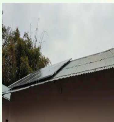
Fig 63. Solar hybrid plant for minimal processing unit 3KVA, single phase, 50 Hz capacity
